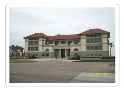
The U.S. Federal Building is located on Shoreline Drive in Corpus Christi, Texas. The building was constructed in 1997 and is generally comprised of structural steel framing. The roof consisted of two types of construction including a low-sloped modified bitumen roof and steep-sloped clay S-shaped tile roofs. Leaks were experienced in the tile roof areas almost since original construction.
