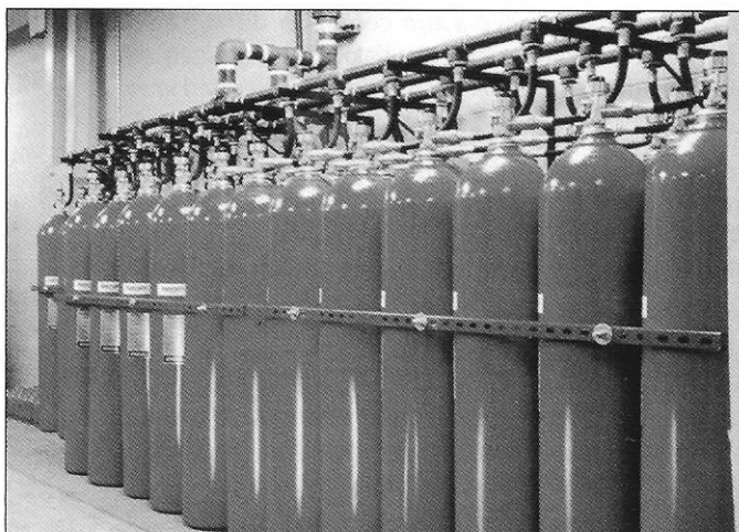
Figure 4 Inergen system
