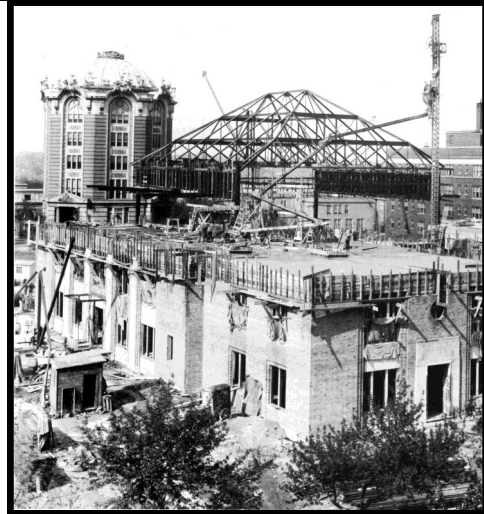
Shaare Emeth under construction in 1931 >
