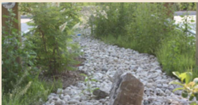
A bioswale captures stormwater run-off from the parking lot.
