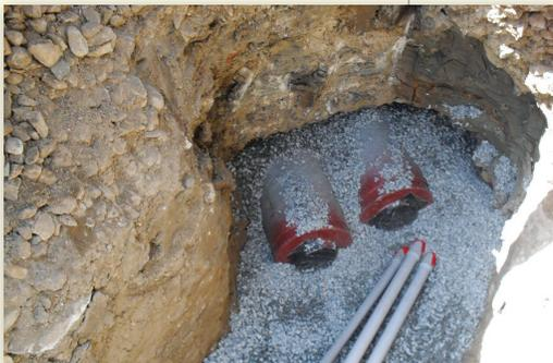
*Due to the proximity of underground steam lines, OmegaFlex recommended the use of an INSUL-TEK<sup>®</sup> 400 HT Composite System to provide for additional heat protection up to 400F for the DoubleTrac Nylon 12 jacket. (pictured above)*
