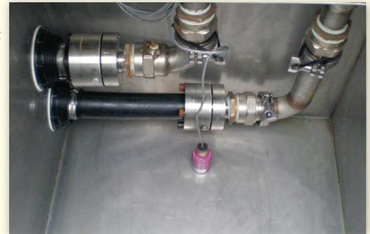
*The new DoubleTrac corrosion resistant Stainless Steel fitting was used for easier assembly in the sump! This fitting provides a metal to metal seal and is field attachable.*
