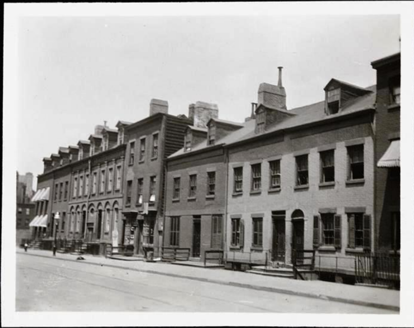
The Charlton-King-Vandam Historic District encompasses the remains of what was once much a larger neighborhood of townhouses extending five blocks from MacDougal Street to the Hudson River. These homes, on the north side of Charlton, between Varick and Hudson, were demolished in 1924 and replaced by commercial buildings including a garage.
