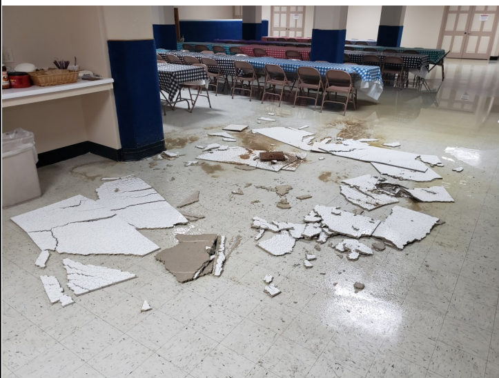
Dining Room Ceiling Damage caused by a broken drain line and repaired by our volunteer work group.
