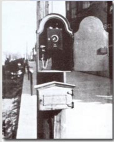
Figure 1. One of Oakland's original call boxes
