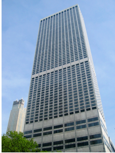
Water Tower Place (1975) Chicago, IL 859 feet tall
