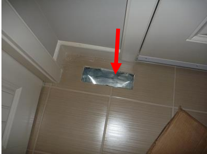
Next to garage man door
