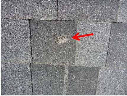
Above garage entrance
