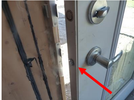
Rear man door in basement
