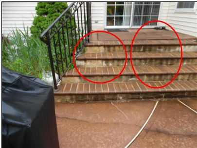
2.6 Item 3(Picture) Area of cracks in rear steps
