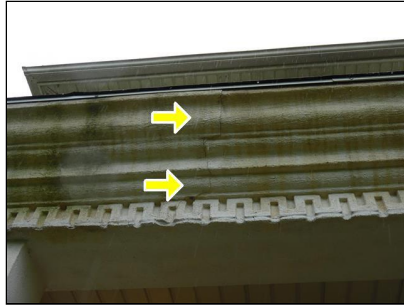
2.0 Item 2(Picture) Cracks in EIFS- Above front entry
