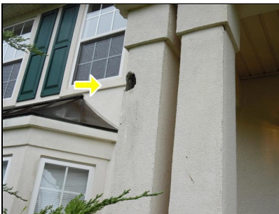
2.0 Item 4(Picture) Hole in EIFS column
