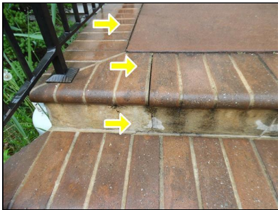
2.6 Item 1(Picture) Cracks in steps
