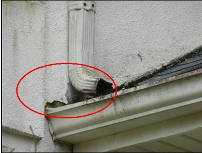
2.0 Item 1(Picture) Hole in EIFS- Right front wall
