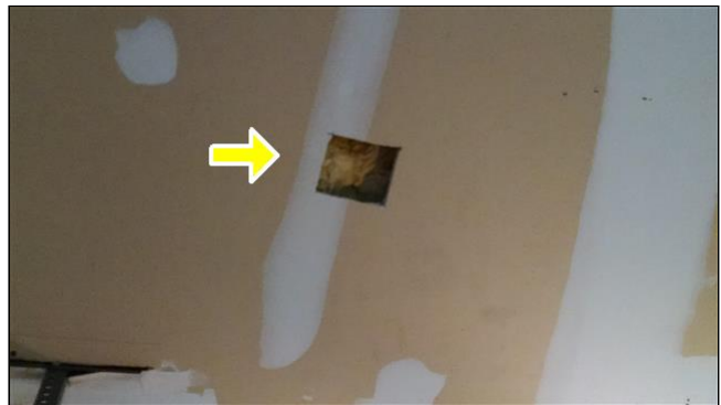
3.7 Item 2(Picture) Holes in drywall on ceiling
