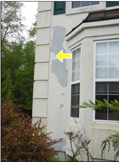
2.0 Item 5(Picture) Final coat on EIFS peeling- left front side of house
