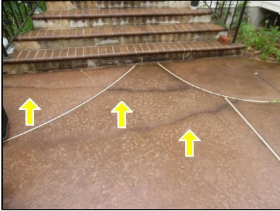
2.10 Item 1(Picture) Cracks in concrete patio
