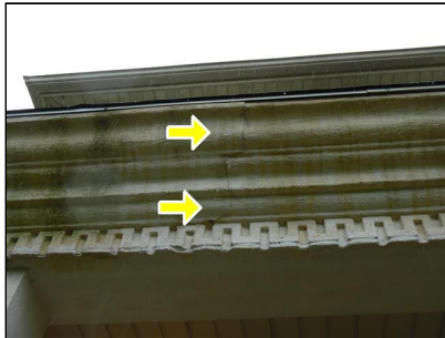
2.0 Item 2(Picture) Cracks in EIFS- Above front entry
