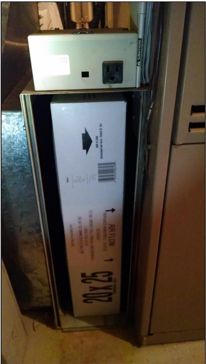
11.4 Item 2(Picture) Disposable filter in cabinet where OEM filter should be
