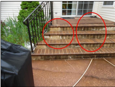
2.6 Item 3(Picture) Area of cracks in rear steps
