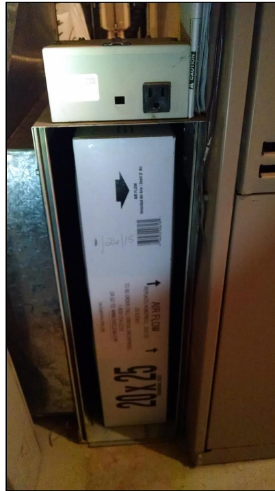
11.4 Item 2(Picture) Disposable filter in cabinet where OEM filter should be
