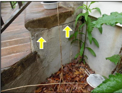
2.6 Item 2(Picture) Cracked parging on right side of rear steps
