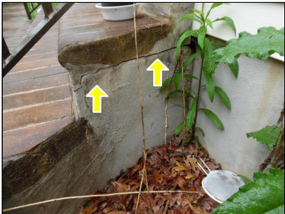
2.6 Item 2(Picture) Cracked parging on right side of rear steps
