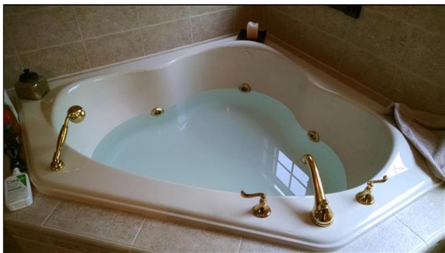
14.3 Item 2(Picture) The jacuzzi jets would not operate
