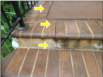
2.6 Item 1(Picture) Cracks in steps
