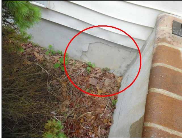
5.0 Item 1(Picture) Paint is peeling on exterior foundation wall
