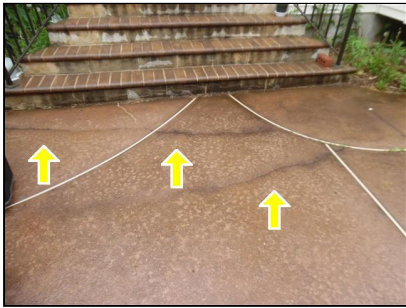
2.10 Item 1(Picture) Cracks in concrete patio
