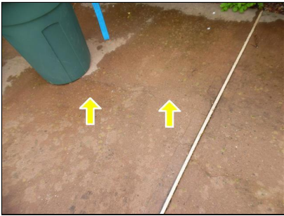
2.10 Item 3(Picture) Crack in concrete patio
