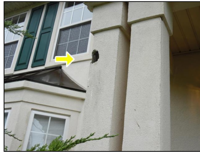
2.0 Item 4(Picture) Hole in EIFS column
