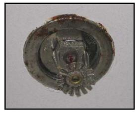
Figure 3 – Corroded Sprinkler Escutcheon Plate
