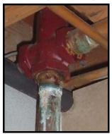
Figure 5 – Corroded Bracket Bolt
