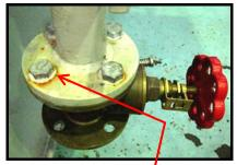
Figure 4 – Corroded Bolts
