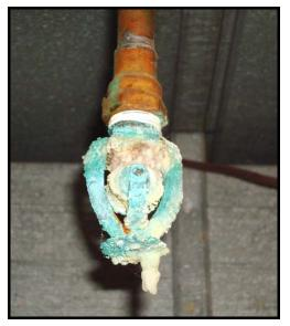
Figure 2 – Corroded Sprinkler
