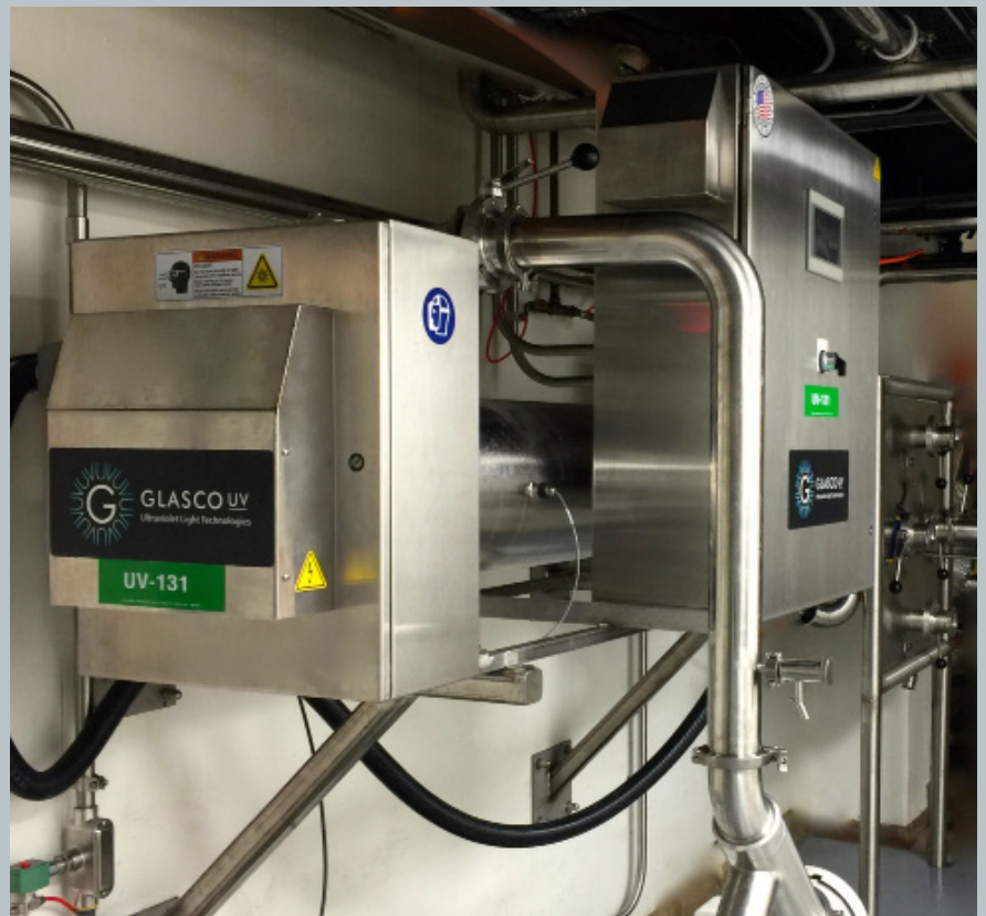
Lamp cooling shrouds are integrated on to each end to provide optimum UV output and cool operating temperature.
