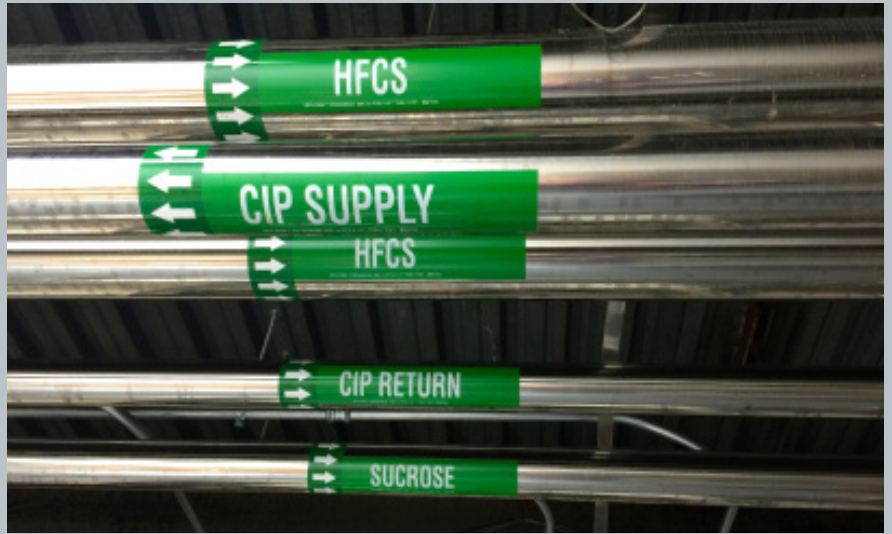
Sanitary piping for Sucrose, HFCS and Clean in Place. The UV system is manufactured from 316L electropolished stainless steel.
