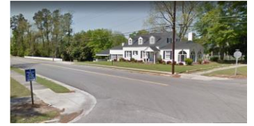
▲ Example of No ADA Transition Pad (Cameron Rd & 1 st Street)
