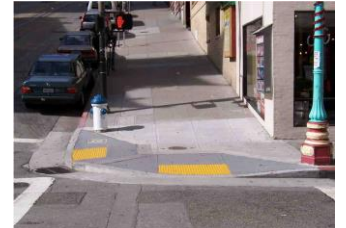
▶ Good design - wheelchair access at intersection & crossing at both roadways
