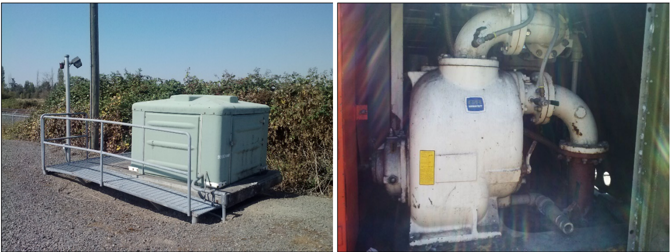
Figure 2-6. Transfer Pump Station Exterior (left) and Pumps Inside (right)
