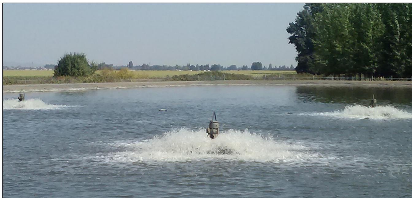
Figure 2-5. Treatment Lagoon Aeration
