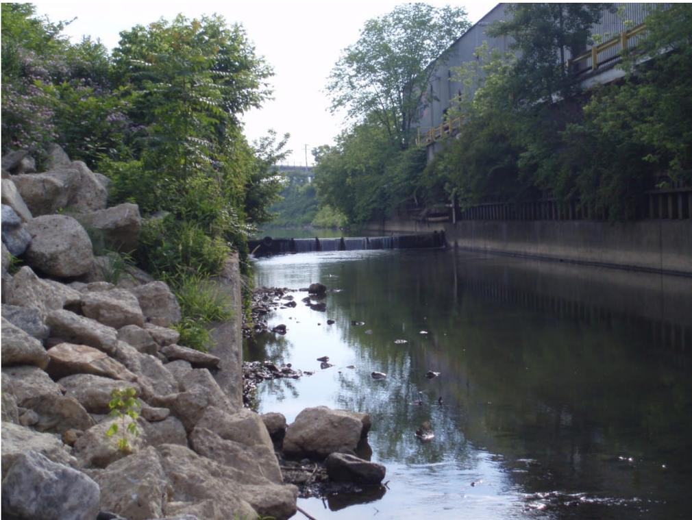
*Looking upstream at the former Barnsteel dam from under the General Butler bridge, as it appeared before its late 2009 removal. Note the long stretch of concrete and steel siding. A busy railroad line is on the left of the picture 25 feet above the creek.*
