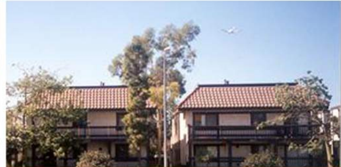
Watts/Athens Preservation Apts. Los Angeles, CA
