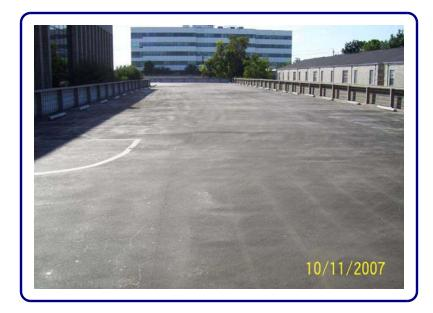
The parking garage adjacent to the Office Building at 9900 Westpark is a 2-level structure comprised of structural steel columns and beam framing with an elevated cast-in-place concrete deck on metal form deck supported by open-web steel bar joists. The elevated deck encompassed approximately 38,100 square feet with an access ramp encompassing approximately 1,100 square feet. CMU walls and metal panel cladding occurred along the perimeter of the garage.
