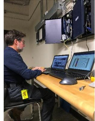
Retuning the BAS in commercial buildings helps to ensure maximum energy efficiency and comfort for building occupants. Although a poorly tuned control system can maintain comfort, it may do so at a high energy cost while compensating for undetected operational inefficiencies.
