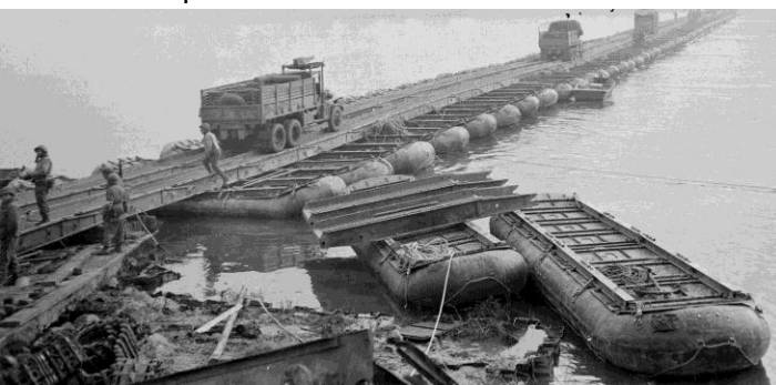
M2 Treadway Bridge in Europe.
