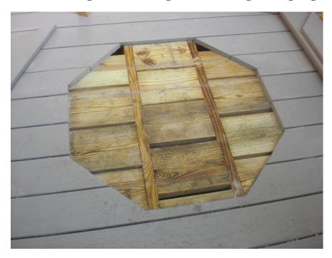
Install inlay and secure with color matched screws or Cortex screws with plugs
