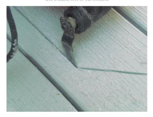
Remove decking...Note blocking installed during framing stage
