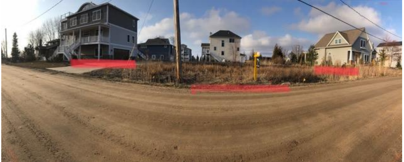
Photo: The north side of Beach where newer homes have built of the grade without regard to the effect of water runoff on neighboring properties and roads. Space between houses approximately 100'.
