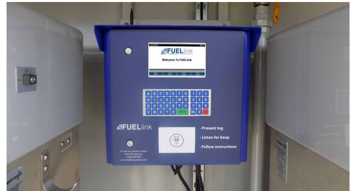
- Wall Mounted Fuel Management System
