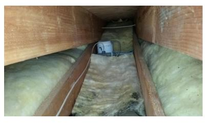
A safe and effective way of sealing off the recessed lighting from your living area is the use of can light covers. We cover the recessed light with a can light cover and seal it with hand held foam. Since the can light cover is safe from fire hazardous hot bulbs and fixtures we are then able to properly insulate around and over the cover itself.
