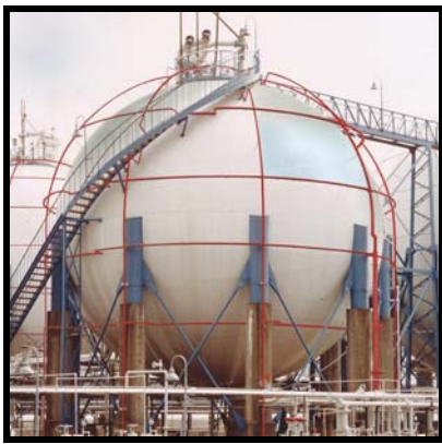
Figure 12 - Correct Sphere Protection
