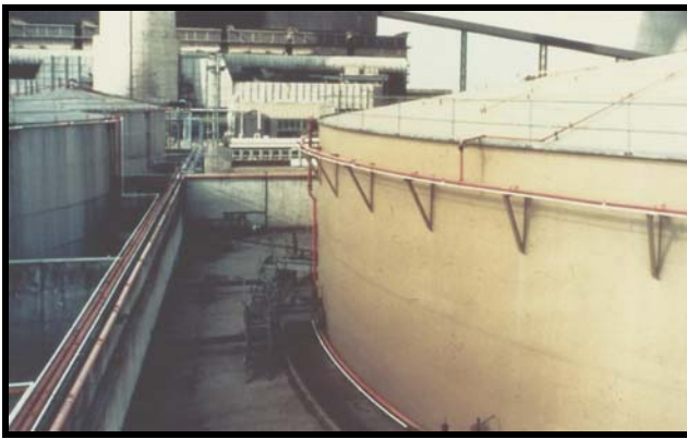
Figure 9 - Protection of a Vertical Cylindrical Tank
