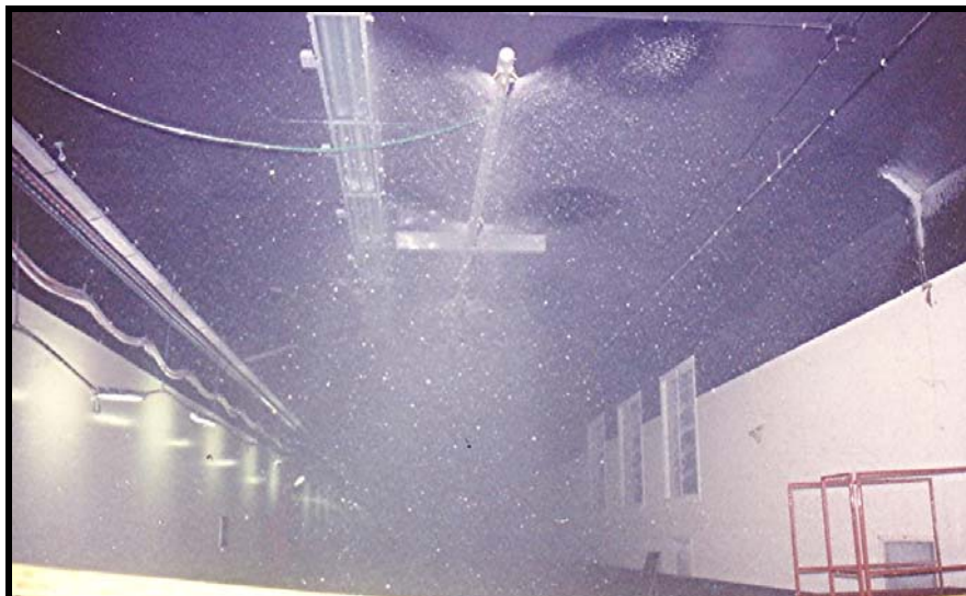
Figure 14 – Sydney Harbour Tunnel Commissioning Test
