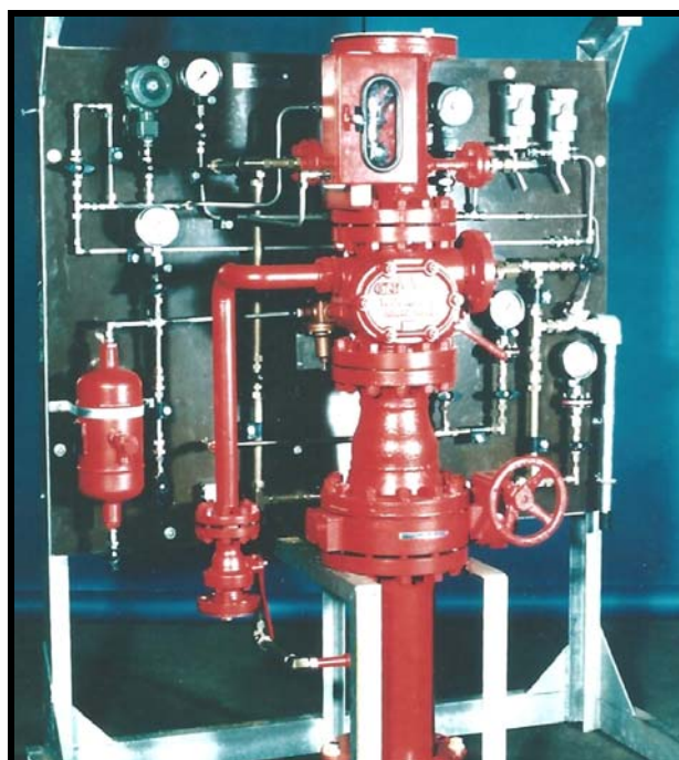
Figure 26 Deluge Valve Skid
