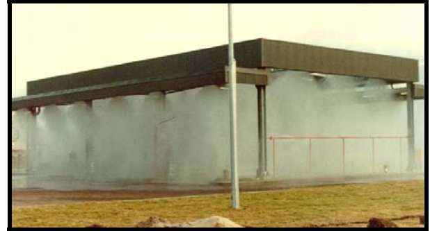
Figure 8 - LPG Tanker Loading Bay
