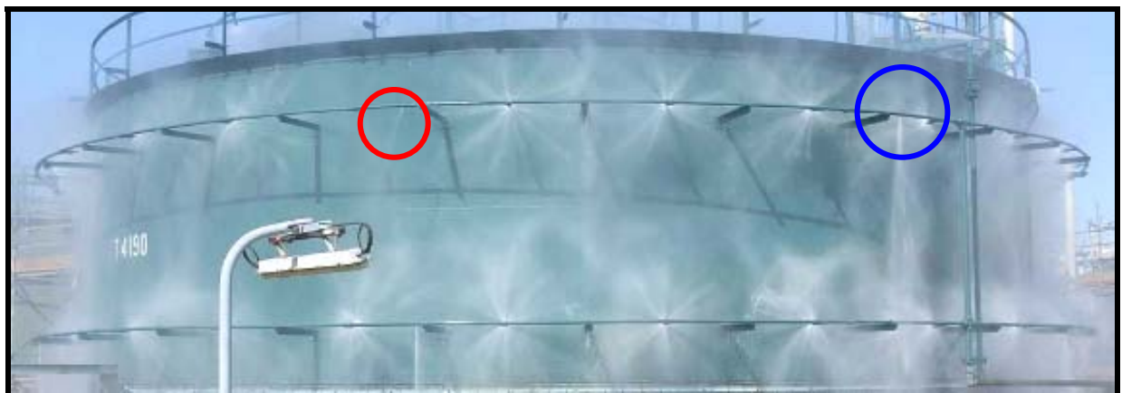
Figure 11 – Floating Roof Tank Shell Protection
