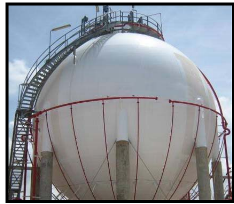
Figure 13 Poor Sphere Protection
