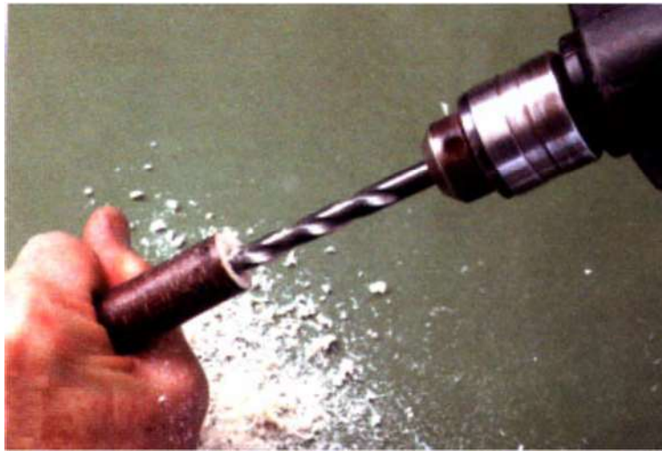
Figure A-1 Drill a Hole
