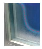
Metal Spacer Condensation builds up because spacers conduct heat and cold.
