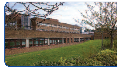
Site of the new Royal Surrey Urology Centre adjacent to St Luke's Cancer Centre
