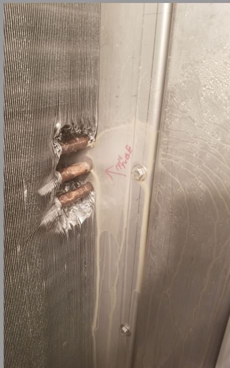
1. Common Chiller Coil Leak
