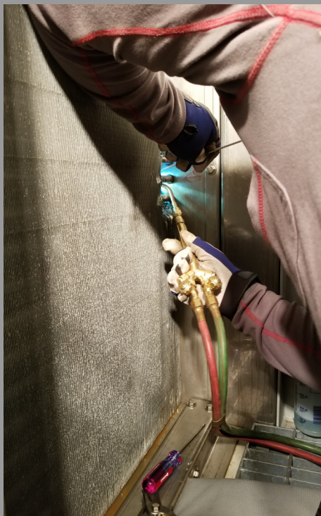
2. Brazing Repair in Process
