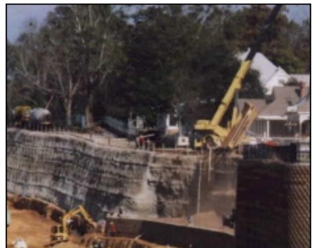
Engineers installed conventional ground anchors and single-bore multiple anchors to stabilize the Mississippi loess. (Photography by Kenneth Bergeron)
