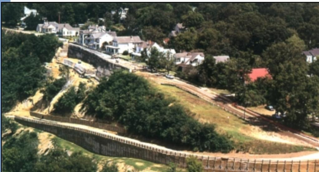
The lower wall is stabilized with soldier piles and anchors, and rises 32 feet and runs for 850 feet; the upper wall has a maximum height of 62 feet and is 450 feet long, and incorporates expanded clay lightweight aggregate.
