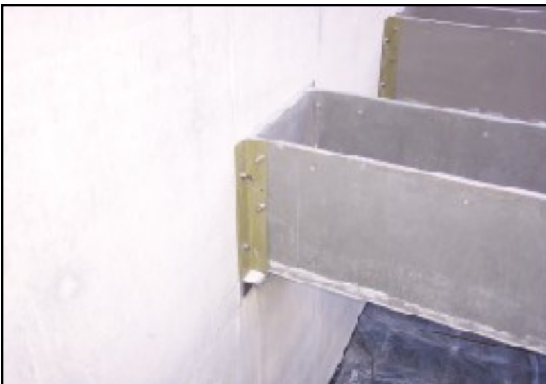
Chalk Bluff, NV trough with blind end and wall saddle mount.
