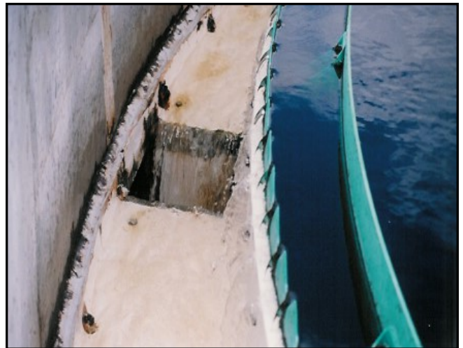
Curved Wall mounted trough with drop out box
