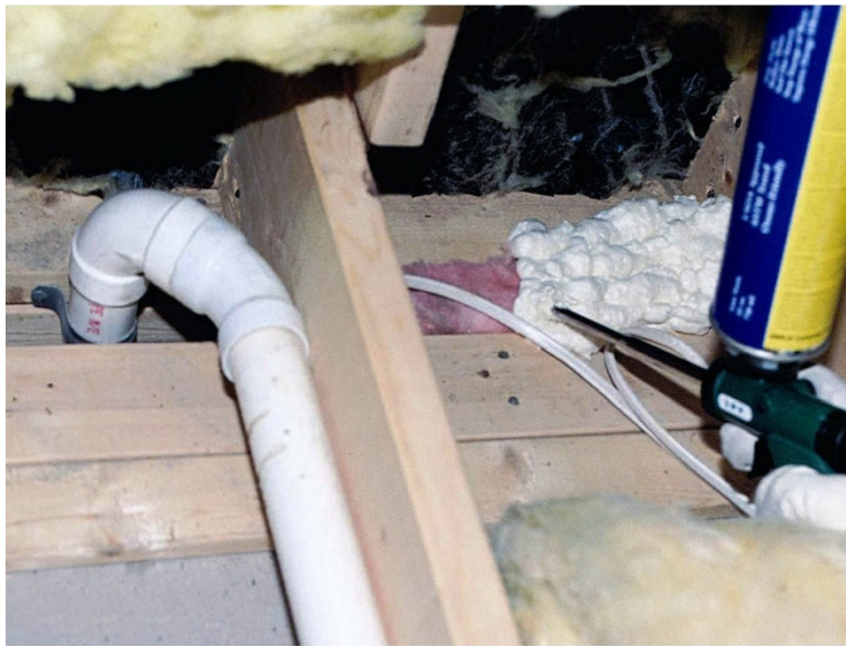
Plumbing Wet Wall Sealed with Fiberglass Batt Backer and 1-Part Foam ( Click to Return to Section )
