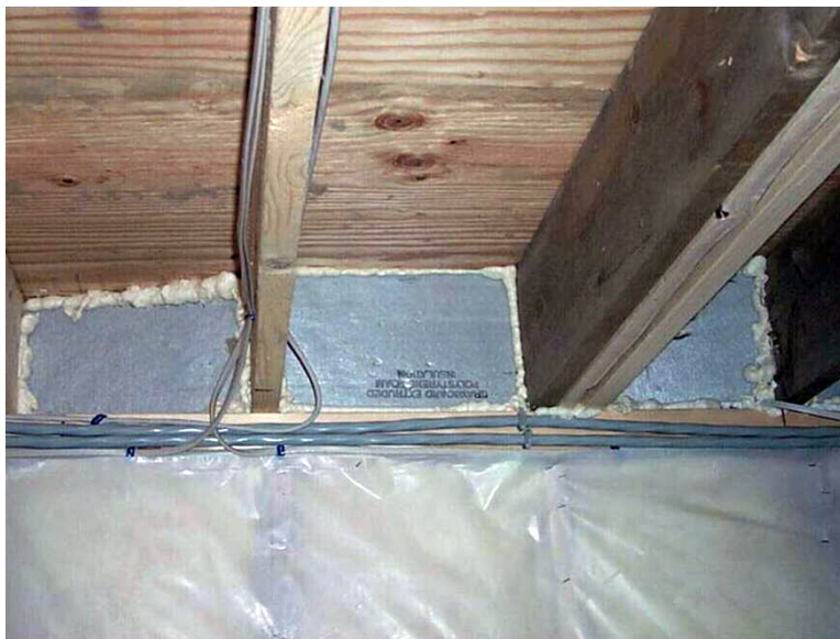
Rim Joist Insulated (and Sealed to Sill) with Foam Board and 1-Part Foam ( Click to Return to Section )
