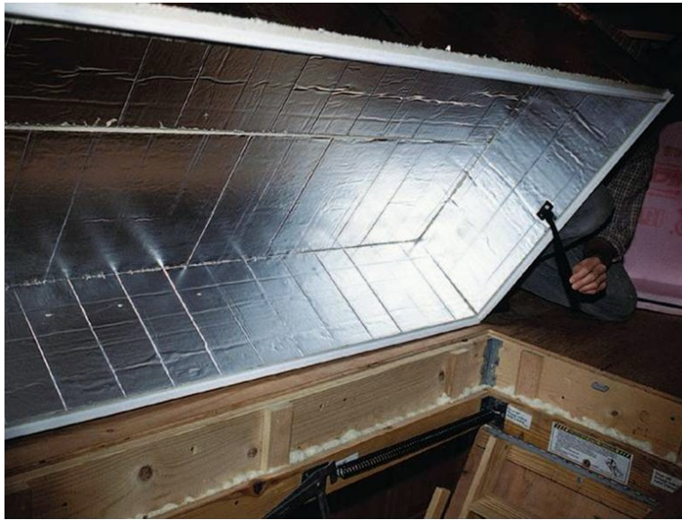
Pull-down Stair Cover ( Click to Return to Section )
