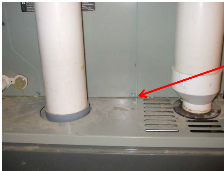
Air Handler Sealed with Silicone Caulk ( Click to Return to Section )
