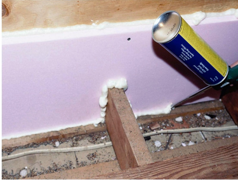
Knee Wall Transition Sealed with XPS and 1-Part Foam ( Click to Return to Section )
