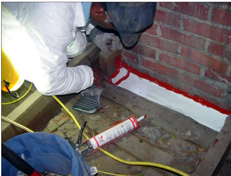
Chimney in Attic Sealed with High-Temp Caulk and Metal Flashing ( Click to Return to Section )
