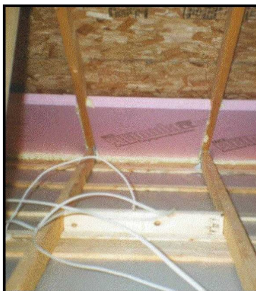
Insulation Wind Wash Baffle ( Click to Return to Section )
