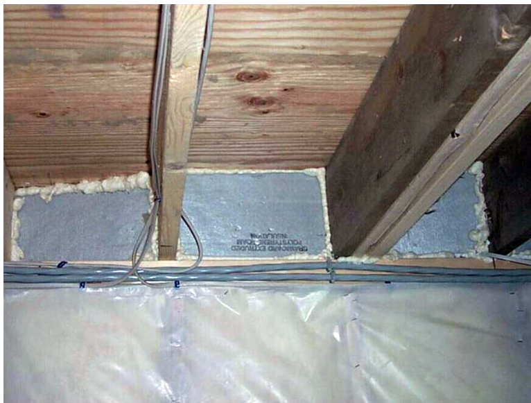
Rim Joist Sealed to Sill (and Insulated) with Foam Board and 1-Part Foam ( Click to Return to Section )
