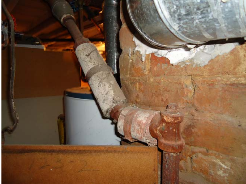
Asbestos Pipe Wrap ( Click to Return to Section )
