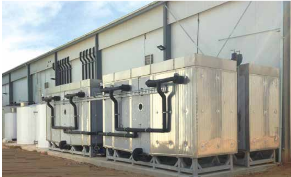
The PCM tanks at Parilla Premium Potatoes in South Australia use a specialised salt-based product.
