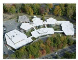
Low-slope roofing membrane installed using low-VOC adhesive and consisting of a SBS-modified bitumen cap sheet and base sheet.
