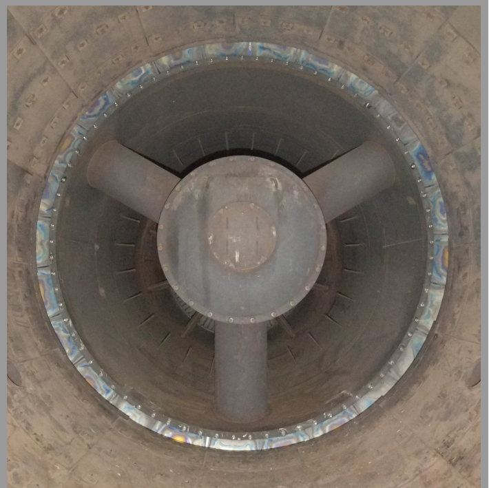
Complete Flex Seal, Gasket, and Hardware Replacement
