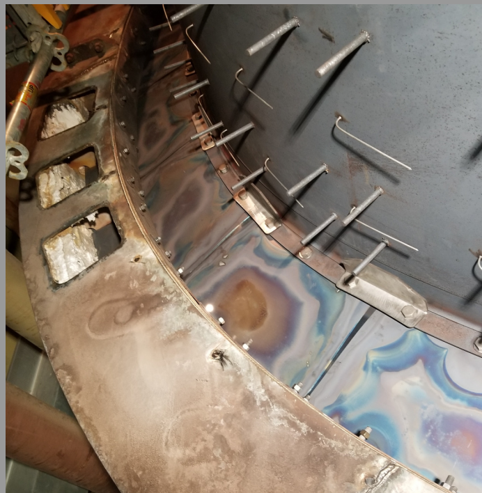
Stud Repair Through Shell Plate
