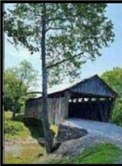
Cabin Creek Covered Bridge Tollesboro, Lewis Co., KY
