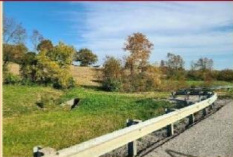
CLOSE-UP AA HWY ENTRANCE
