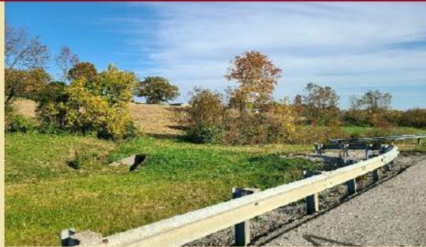
CLOSE-UP AA HWY ENTRANCE
