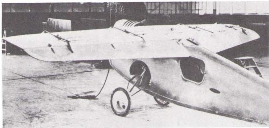
OVERHEAD VIEW shows rods which activated wing flaps, and the gear mechanism. Failure of these linked mechanisms caused racer to drop out of 1920 Gordon Bennett race, after 178-mph qualifying run. (57)
