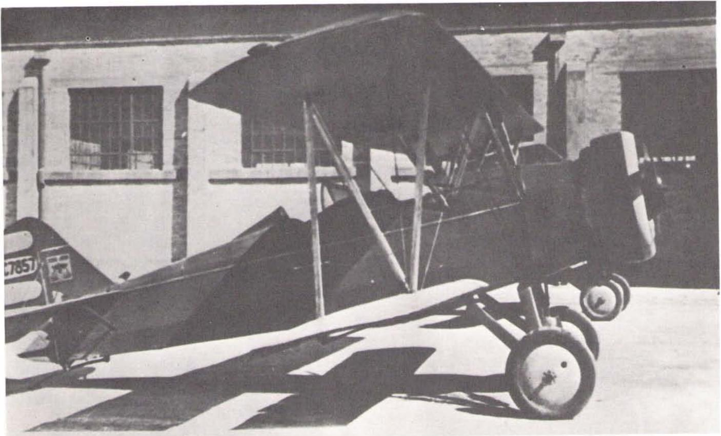
SKYWAY PROTOTYPE was tailheavy, but impressed builders on first flight.
