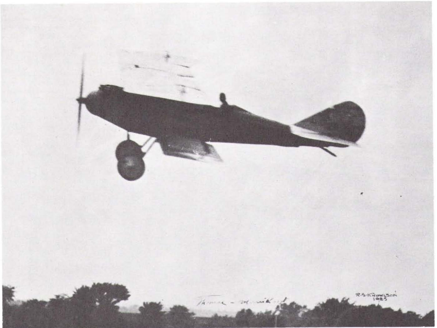
THOMAS-MORSE developed "tail flutter" from poorly arranged elevator wires. Ben sold it.
