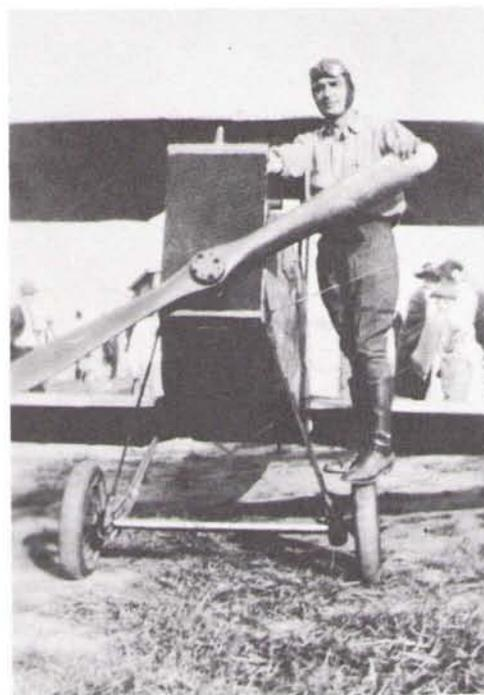
THE BUILDER poses proudly by his bird. Propeller was attached to crankshaft by four bolts — there was no propeller shaft. (38)
