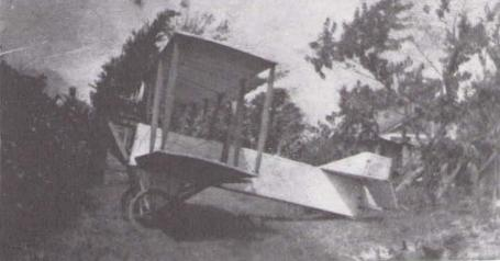
SIDE VIEW is less flattering. Aircraft was all wood construction.
