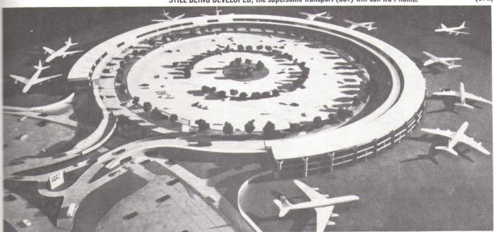
TOPOGRAPHICAL MODEL of KC-I shows unique circular terminal modules.
