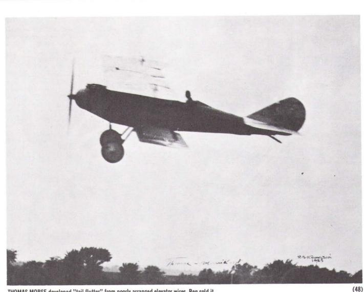
THOMAS-MORSE developed "tail flutter" from poorly arranged elevator wires. Ben sold it.
