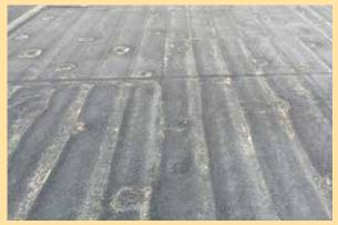
Example of rutting in polyisocyanurate insulation in an adhered EPDM membrane roof system
