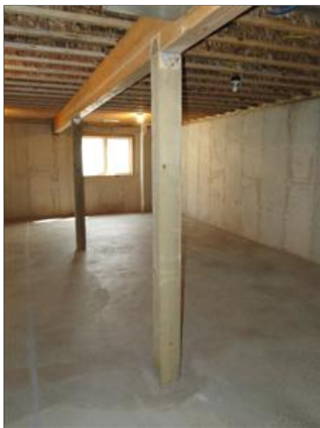
9.1 Picture 1 Wood piers at basement.
