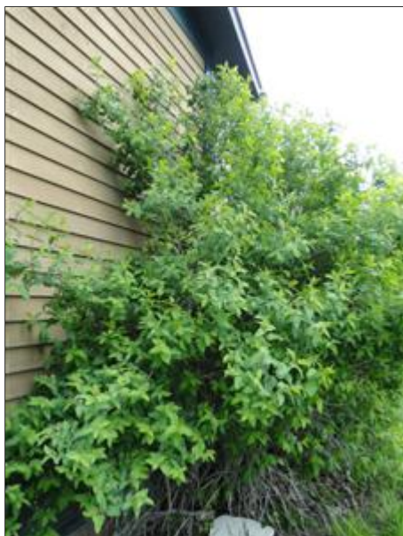
2.1 Picture 8 Trim back vegetation to allow cladding to breath.
