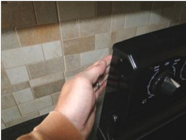
5.13 Picture 1 Oven tips away from wall easily.
