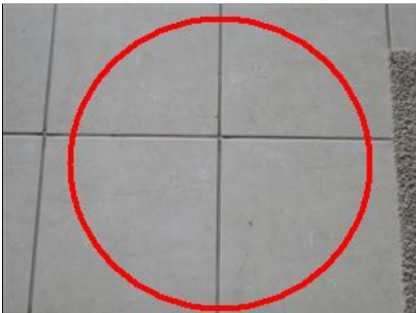
7.2 Picture 1 Tiles sound hollow here.
