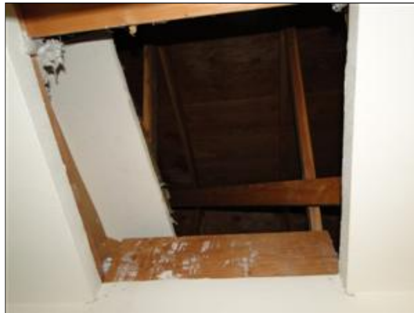
4.0 Picture 1 View of attic access.
