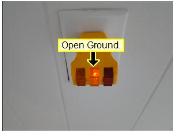
5.5 Picture 1 Outlet east wall open ground.
