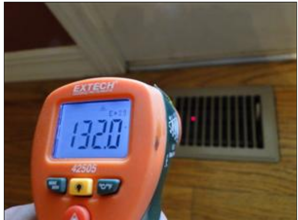
11.0 Picture 4 132 at main floor vents.
