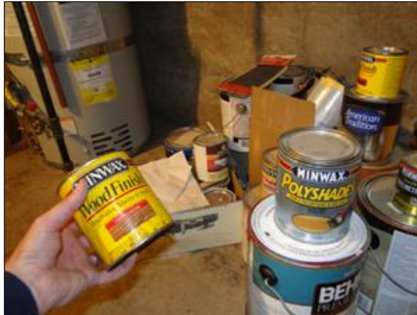
10.5 Picture 1 Paints and stains next to water heater.
