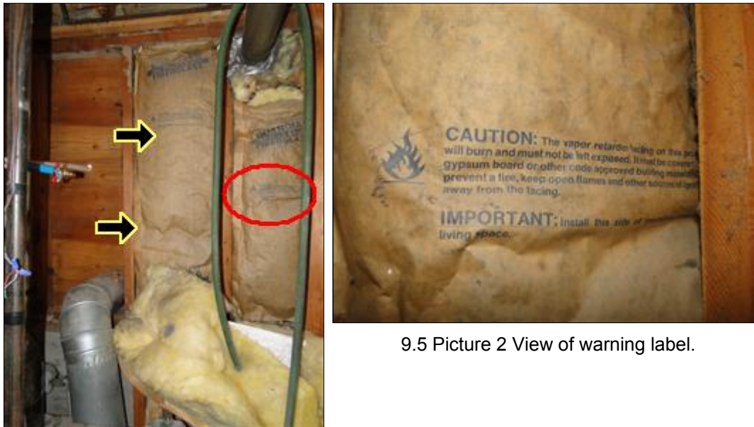
9.5 Picture 1 Kraft back insulation, read warning label.
