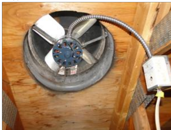
4.3 Picture 1 View of attic fan.
