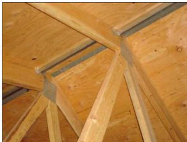
4.2 Picture 1 View of roof structure.
