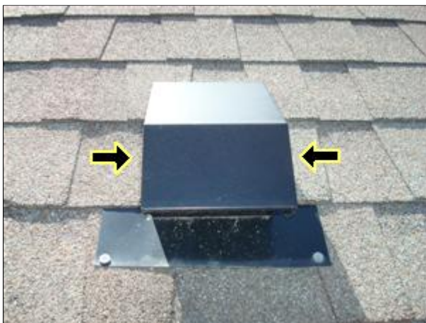
1.2 Picture 2 Look under this vent hood.
