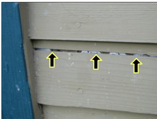
2.1 Picture 2 Split cladding board.
