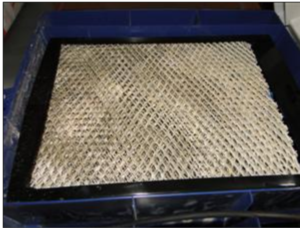
11.0 Picture 7 View of interior pad.
