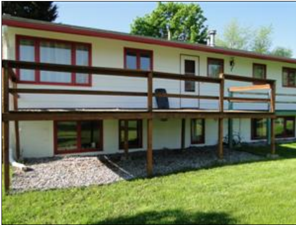
2.4 Picture 1 Over view of deck.
