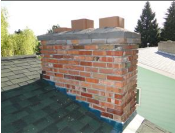
1.2 Picture 4 View of chimney.
