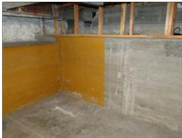
9.0 Picture 1 Masive foundation walls.
