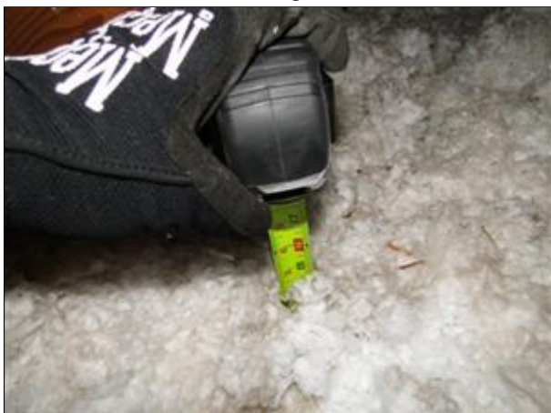
4.1 Picture 1 16" blown in insulation.
