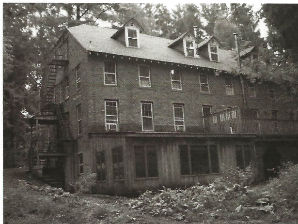
Former dormitory building Camp Midvale, then Weis Center
