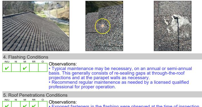
• Exposed fasteners in the flashing were observed at the time of inspection. It is recommend not to have nails driven through this flashing; may cause water intrusion into the attic.
