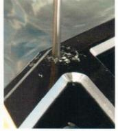
4. After holes are made use provided hardware to install accent plate (polished hardware).
