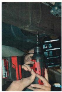
**17.** Insert sinch nut into frame using the supplied tool. Tighten nut down using a 3/4" socket and 13/16" wrench.
