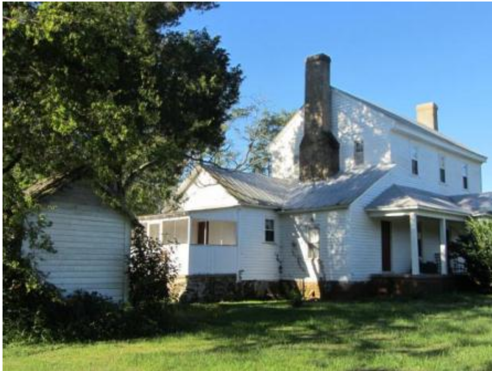
Figure 23. NCDOT Survey #9, Andrew Gibson Farm (GF-0585, 7282 Burlington Road, Guilford County), northeast elevation, looking south-southwest; wellhouse is on the left.
