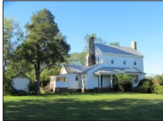
NCDOT Survey #9, Andrew Gibson Farm (GF-0585), looking southwest.
