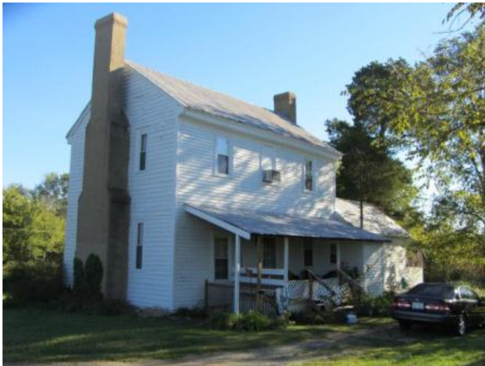
Figure 25. NCDOT Survey #9, Andrew Gibson Farm (GF-0585, 7282 Burlington Road, Guilford County), south (rear) elevation and west gable end, looking northeast.
