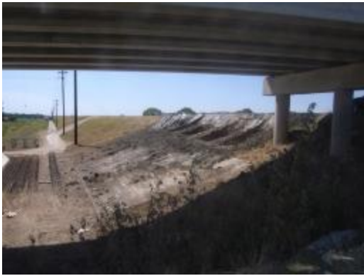
Levee raises and improvements
