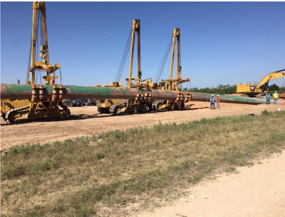
Pipeline construction in the Texas Hill Country. Photo: RRC
