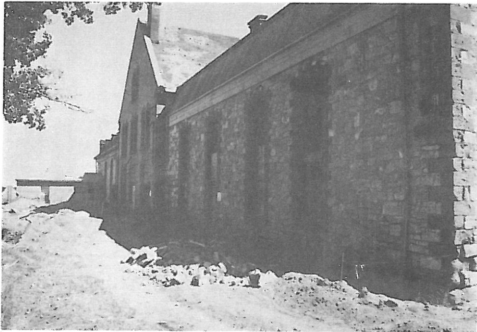
Figure 2: Contemporary view of west side, Wyoming Territorial Prison building, showing north wing kitchen addition.
