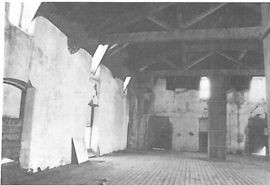
Figure 3: View of north wing loft area inside main prison building.
