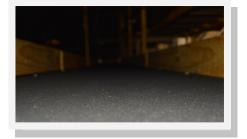
(G). <u>Non-Skid Deck Coating</u> <u>for All Platforms</u>: this is an optional feature that adds a Non-Skid Surface to the Platforms. This is a product that was developed with Herculiner Polyurethane Coatings, the same product used for bed liner coatings for pick-up truck beds "<u>Optional Feature</u>"
