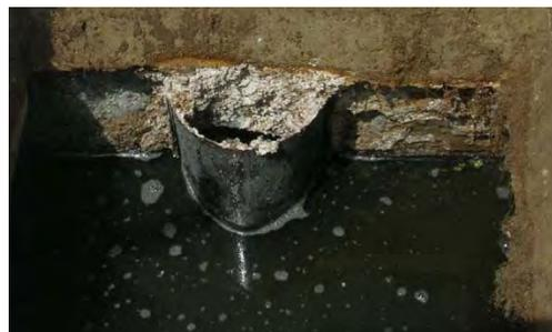
Illustration 1 Concrete Corrosion around Outlet Baffle
