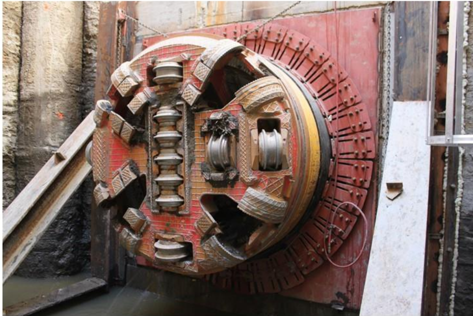
Exit Ring and Seal, 82" OD, Steel Pipe
